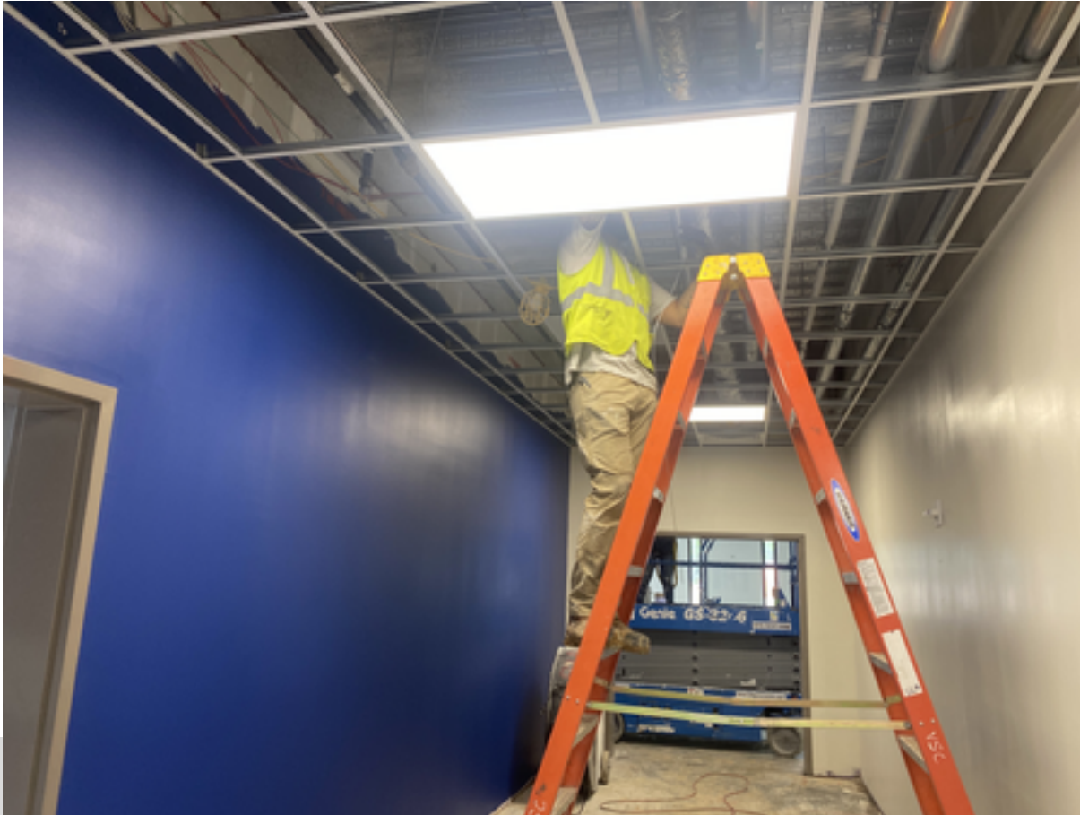
Interior lighting install in new building
