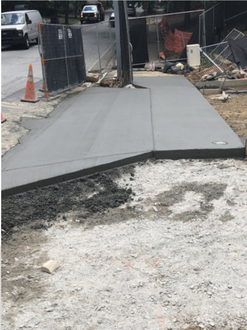
Concrete apron install
