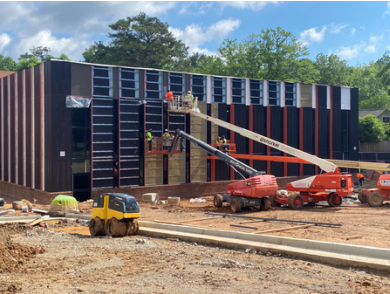
Metal wall panel install
